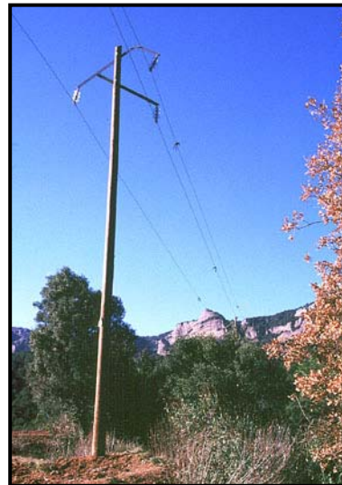
Figure X: Save pylon with a “Canadian” cross arm configuration (Sant Llorenç del Munt, 2002).
