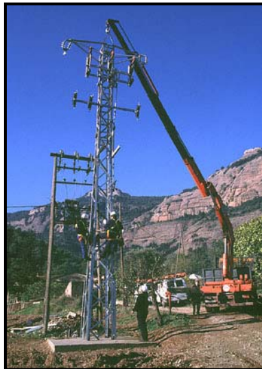
Figure IX: Application of corrective measures against bird electrocution. Substitution of a dangerous pylon (Sant Llorenç del Munt, 2002).
