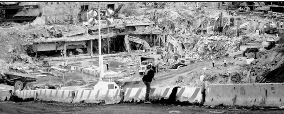
(Above) Fall protection--Jersey (cement) barricades along the Tully Roadway protected vehicle operators and recovery workers from fall injuries.
