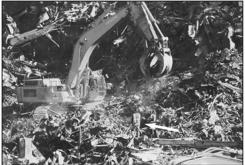
(Above) Lone spotter (debris removal observer) wore reflective vest (arrow) and stayed 50 feet from the operating radius of a demolition grappler.
